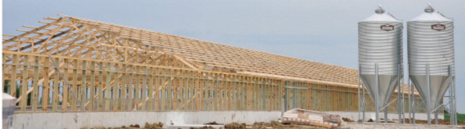
Image provided by New Modern Construction
