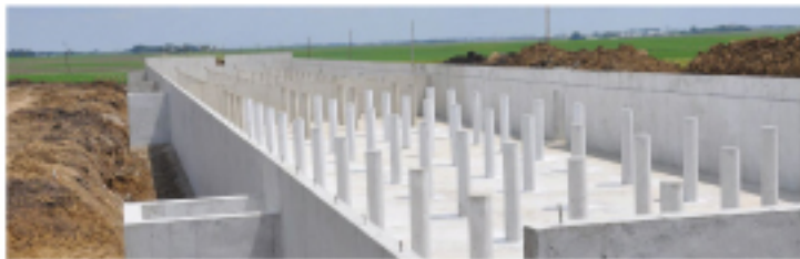
Image provided by New Modern Construction
